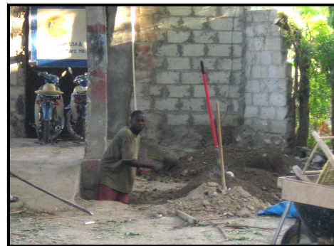
Construction of the solar panel support gets underway.
